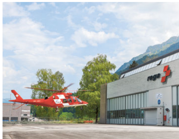
The infrastructure of the Wilderswil base has been upgraded.
