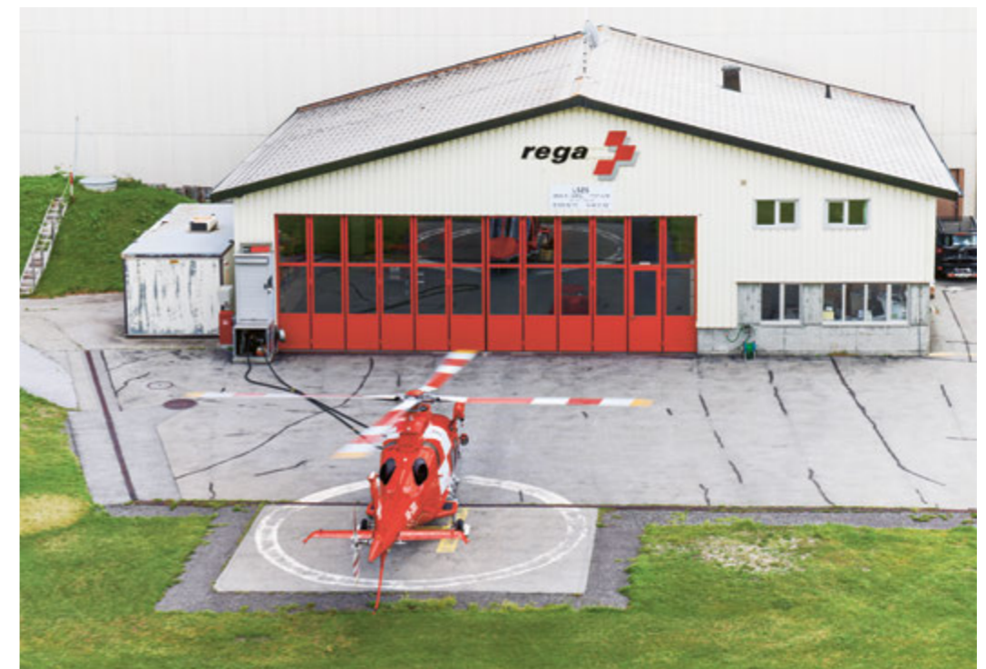
At Rega's highest-lying helicopter base, the over 45-year-old building is being replaced by a brand new one.
